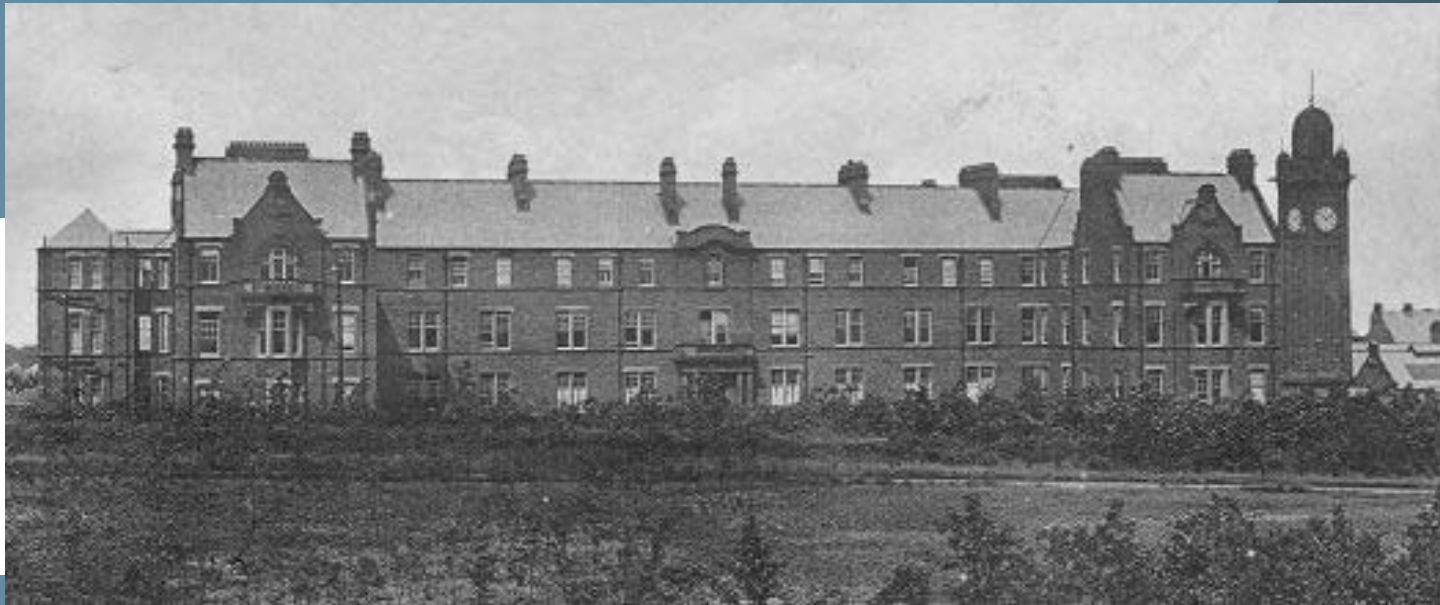
Glasgow Stobhill hospital (1904-2009)
